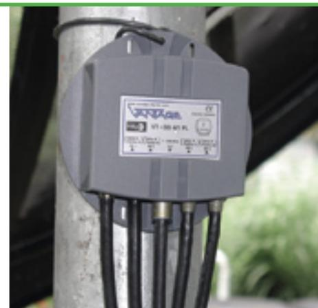
**DS 4/1 PL switch connected to the same 10-foot dish plus two additional antennas**
